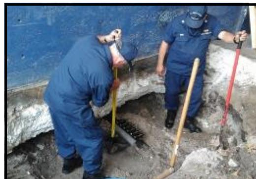
**Alfredo Schwartz (left) and Humberto Jahen (right) pound down the sand around the stainless steel repair of the water line to stabilize the dirt before the line is covered.**
