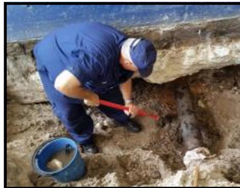
**Julio Garcia digs under “leaky” fire suppressant main line at Air Station Miami in preparation for the repair.**
